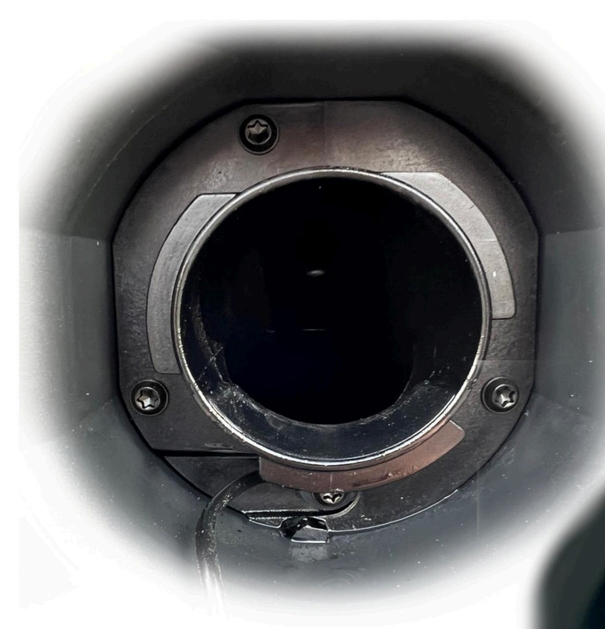
Twist the supplied adaptor ring onto the neck making sure the seal is in place first & until its tight, secure with the two screws (No Drilling Required)
